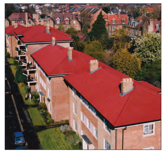
Boldroll ridge to eaves sheets can be fixed to a steel/timber sub-structure as in this flat to pitched roof conversion.
