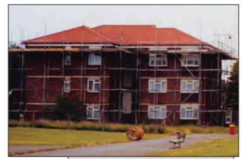
Boldroll ridge to eaves tile effect roofing sheets offer improved structural integrity over traditional materials, making them a popular choice for areas with high levels of vandalism.
