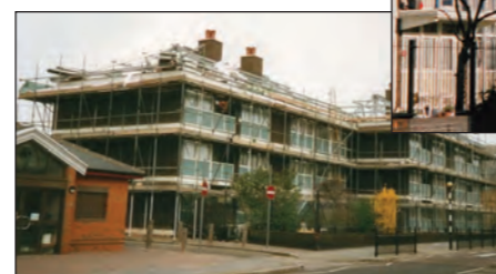
The Pantile 2000 ridge to eaves sheets can be fixed to a steel/timber sub-structure, as in this flat to pitched roof conversion.
