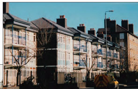
The Pantile 2000 ridge to eaves sheets can be fixed to a steel/timber sub-structure, as in this flat to pitched roof conversion.
