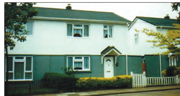
The Pantile 2000 fast-track roofing system considerably reduces time on site, keeping disturbance to a minimum.
