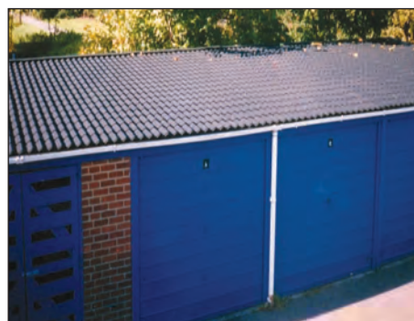
The rigidity of the Pantile 2000 lightweight sheets permit direct fixing to reinforced concrete purlins with no additional support required.
