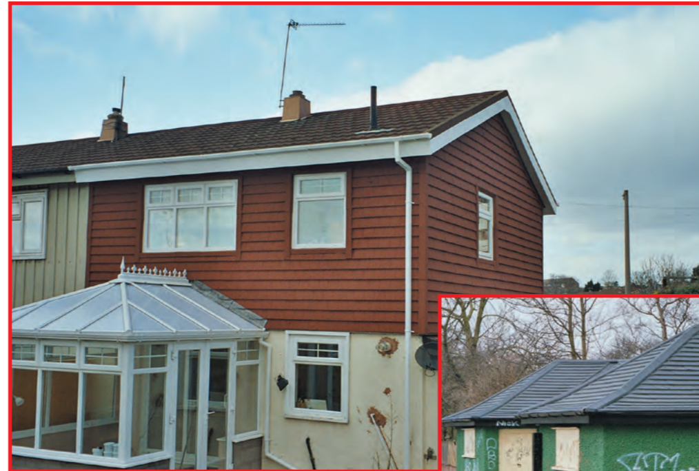
The Plain Tile's aesthetic characteristics permit its use in a wide variety of applications including vertical cladding.
