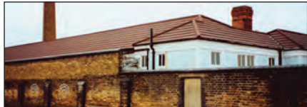
Re-roofing on traditional houses in Slate 2000.
