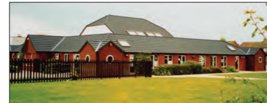
This school project used the 0.9mm thick Slate 2000 because of the high vandalism.
